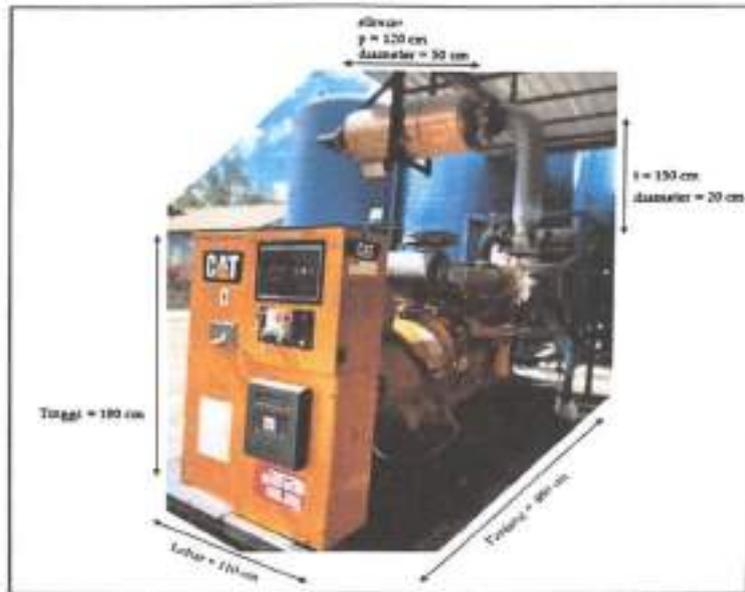
Gambar desain cerobong unit genset Cementing Schlumberger
